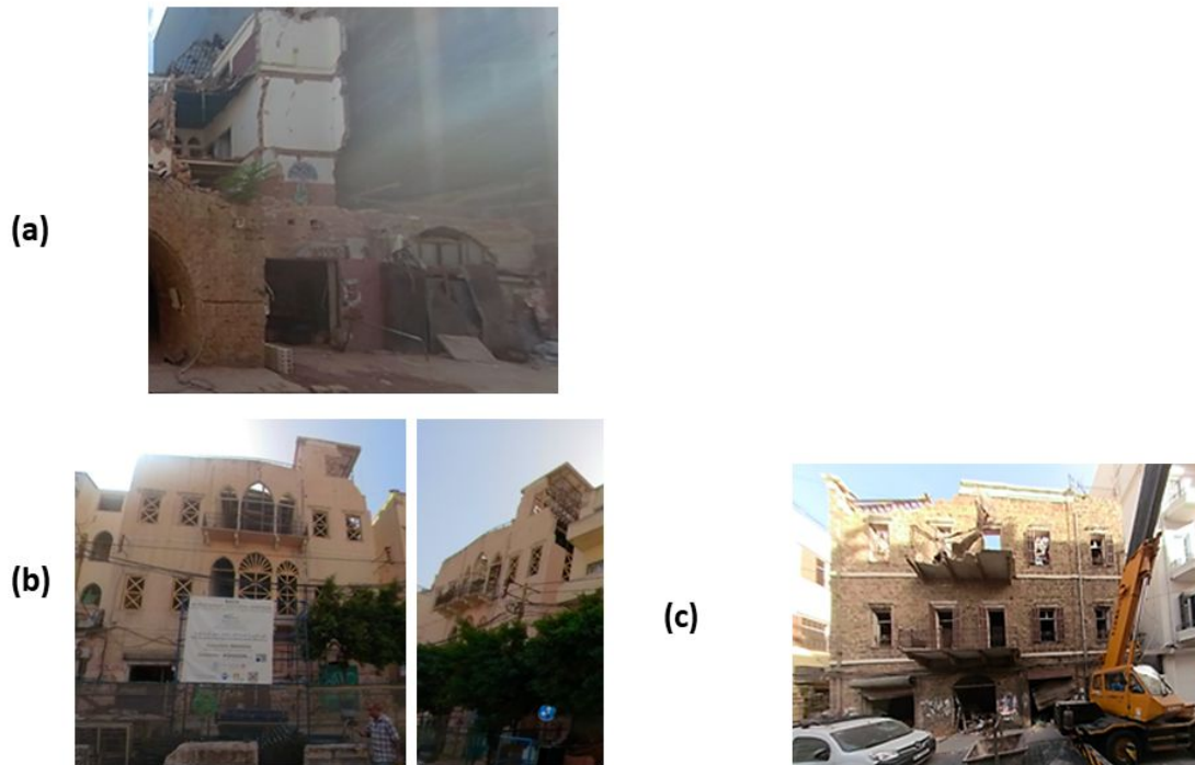
Figure 4.6. Heavily damaged stone masonry buildings classified based on 360 photos: (a) building SM1 (33.8952° N, 35.5202° E), D4-D5; (b) building SM2 (33.8956° N, 35.5223° E), D4; and (c) building SM3 (33.8953° N, 35.5172° E), D3-D4.
