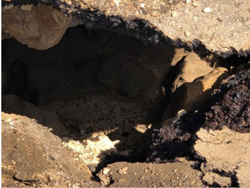
Figure 3.33. Close-up of the void below the asphalted section/pavement (33°54'2.00"N; 35°31'11.36"E).
