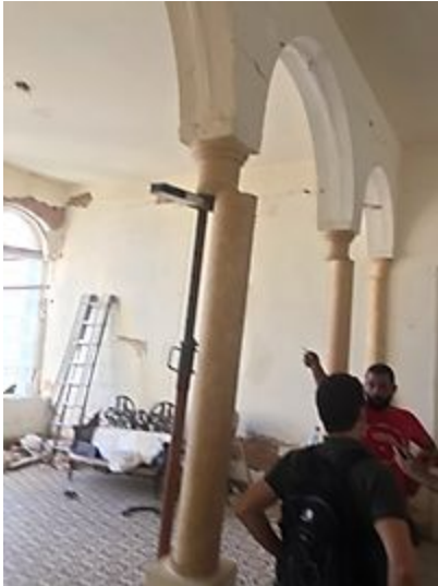
Figure 4.9. Heavily damaged (D3) stone masonry building SM6 (33.8958° N, 35.5192° E).
