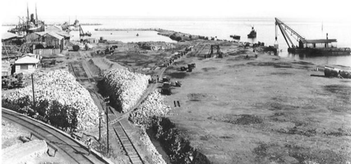
Figure 3.2. Works on the Beirut Port expansion in 1886. Note the cast large blocks, which would then be taken and sunk into position.
