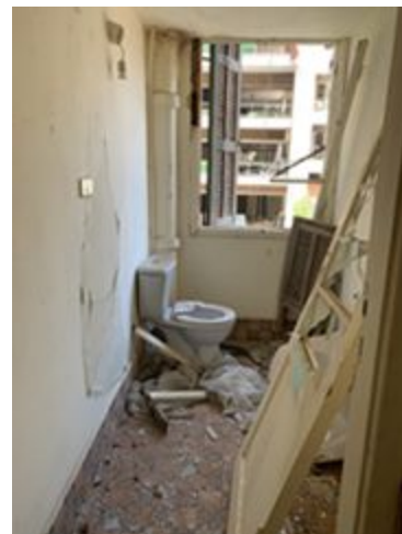
Figure 4.7. Partially collapsed (D4) stone masonry building SM4 (33.8948° N, 35.5161° E).
