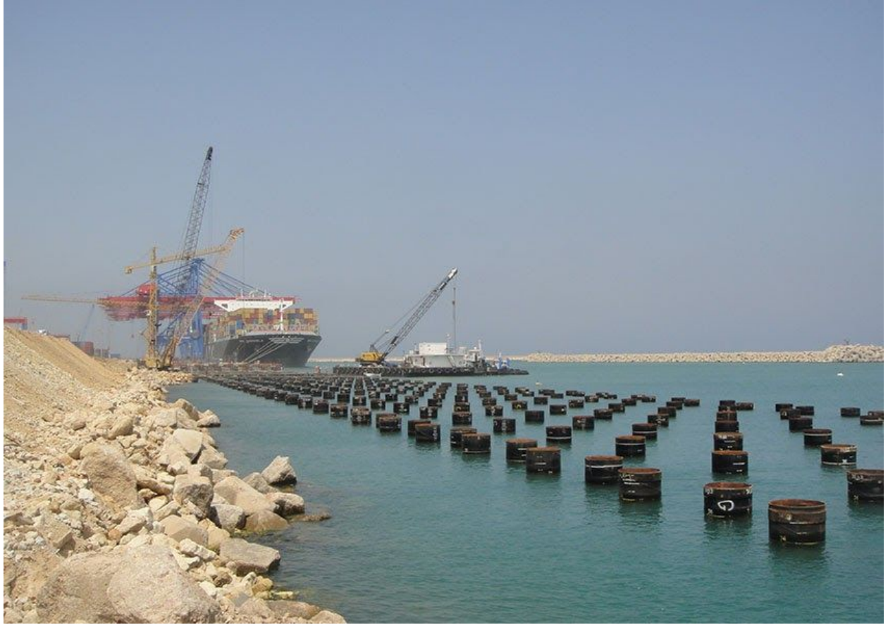
Figure 3.38. Piles driving in Container Terminal portion of Port of Beirut as part of 2011 expansion.
