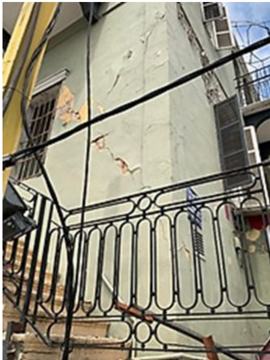
Figure 4.8. Partially collapsed (D4) stone masonry building SM5 (33.8996° N, 35.5260° E).
