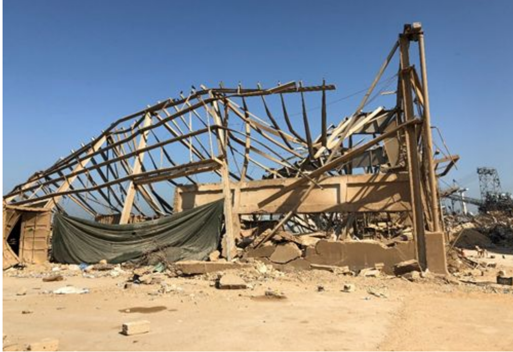
Figure 3.37. Typical damage done to steel structures throughout the Port. All suffered either this level of damage or worse (extent evident in Figure 3.29) ( 33°54'4.23"N 35°31'15.04"E).
