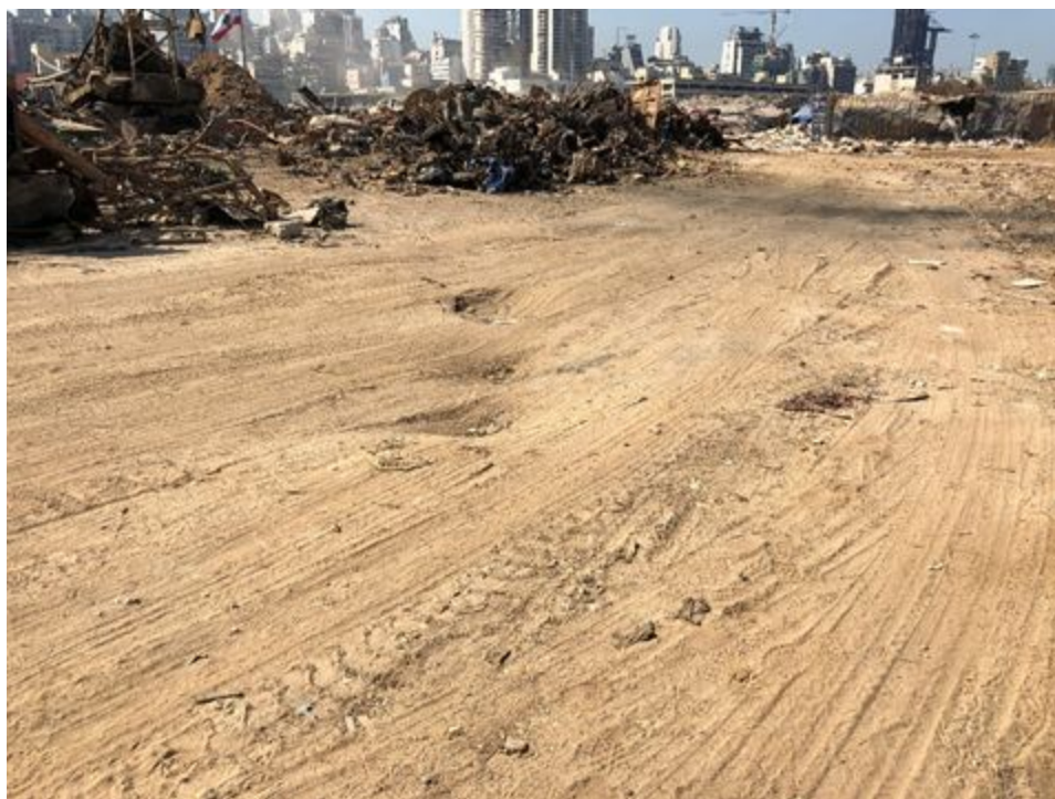
Figure 3.30. Ground deformation and mini-cratering exposed by truck traffic and possible resulting from loosening and/or shifting of the fill below. (33°54'0.86"N; 35°31'9.30"E).
