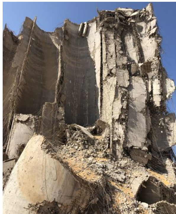
Figure 3.19. Complete failure/crushing of the concrete and collapse of the shell structures ( 33^{\circ}54'6.61''\text{N} ; 35^{\circ}31'5.43''\text{E} ).
