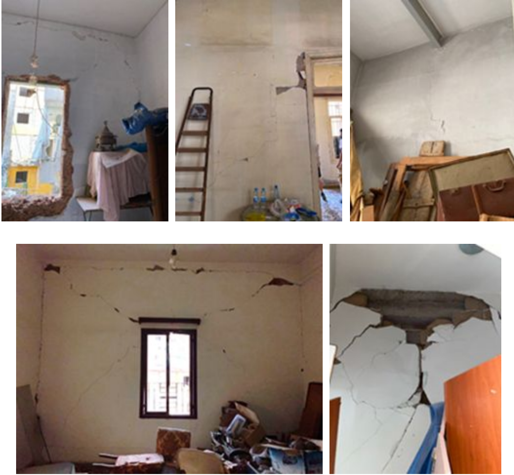
Figure 4.10. Another example of a heavily damaged (D3) stone masonry building SM7 (33.8954° N, 35.5214° E).
