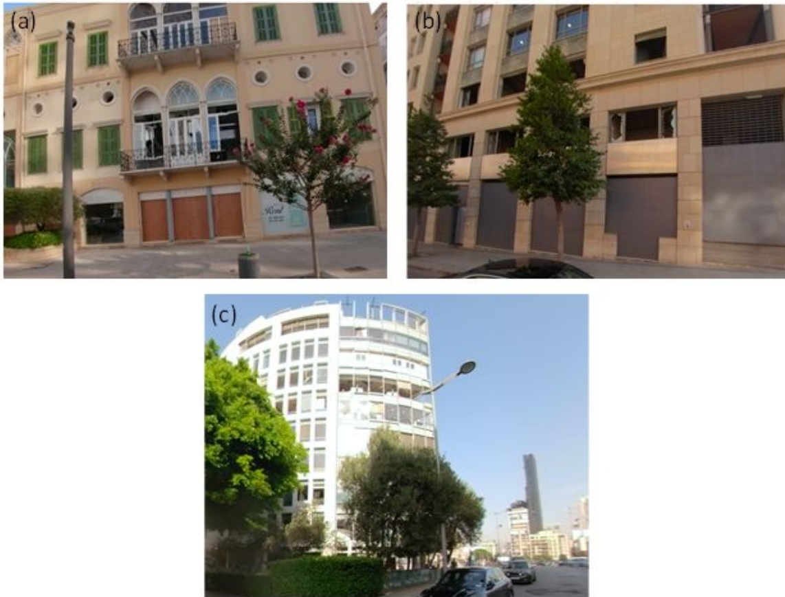
Figure 4.17. Example of façade damage levels (a) Wxx-1: damage to windows only, (b) Wxx-2: damage to windows and frames, and (c) Wxx-3: complete blow-out of frames.
