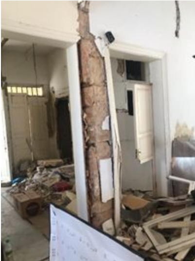
Figure 4.9. Heavily damaged (D3) stone masonry building SM6 (33.8958° N, 35.5192° E).
