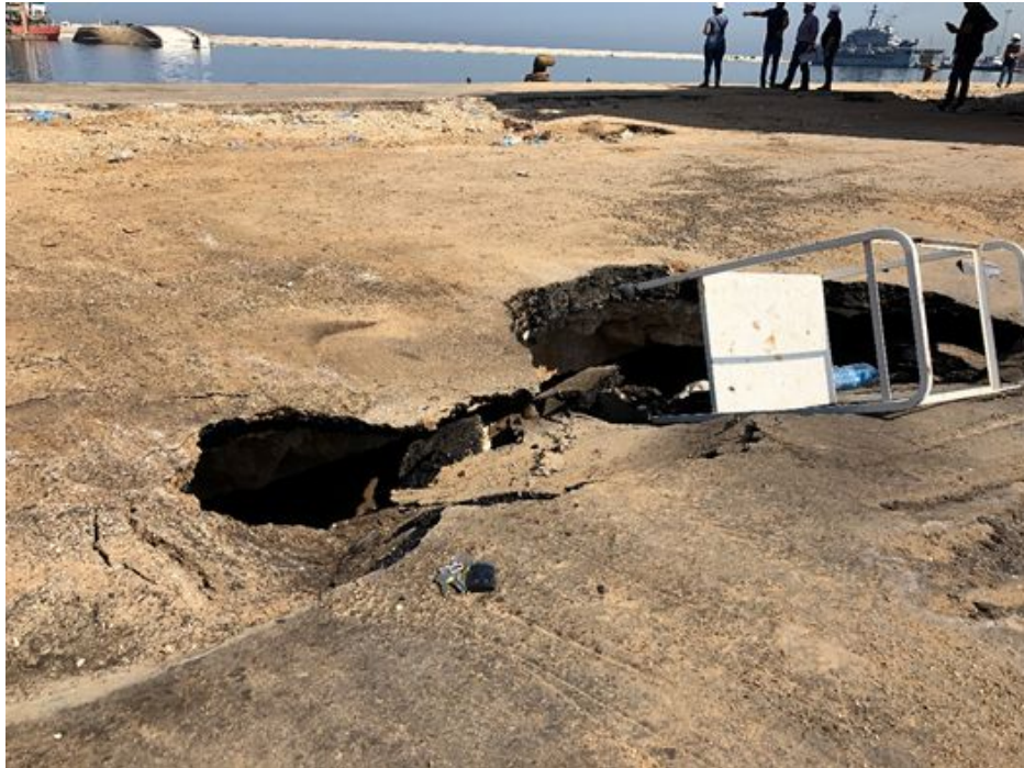
Figure 3.32. Dock along Quay 10. This location was paved. The expression of the ground deformation below the surface was exposed as a result of heavy earth moving equipment. Note the overall downwards settlement from the presumed original quay level ( 33^{\circ}54'2.00''\text{N} ; 35^{\circ}31'11.36''\text{E} ).
