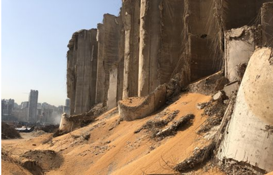
Figure 3.18. Picture taken from the seaside close to Quay 8 looking south towards the city ( 33^{\circ}54'6.97''\text{N} ; 35^{\circ}31'6.54''\text{E} ) . Note the mounds of grain (corn in this case) potentially contributing to structure stability.
