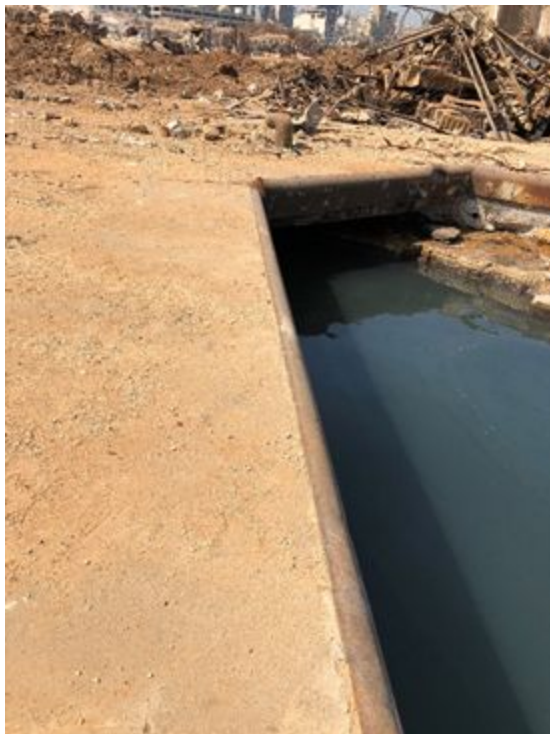
Figure 3.36. No evidence of damage to the western section of Quay 10. Alignment and level of the top quay slab in this section is intact (Location of these images is indicated by the red lines on Figure 3.29) ( 33°54'4.23"N; 35°31'15.04"E).
