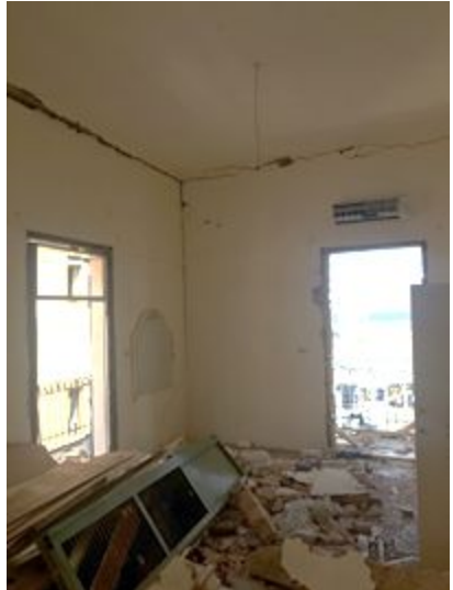
Figure 4.9. Heavily damaged (D3) stone masonry building SM6 (33.8958° N, 35.5192° E).
