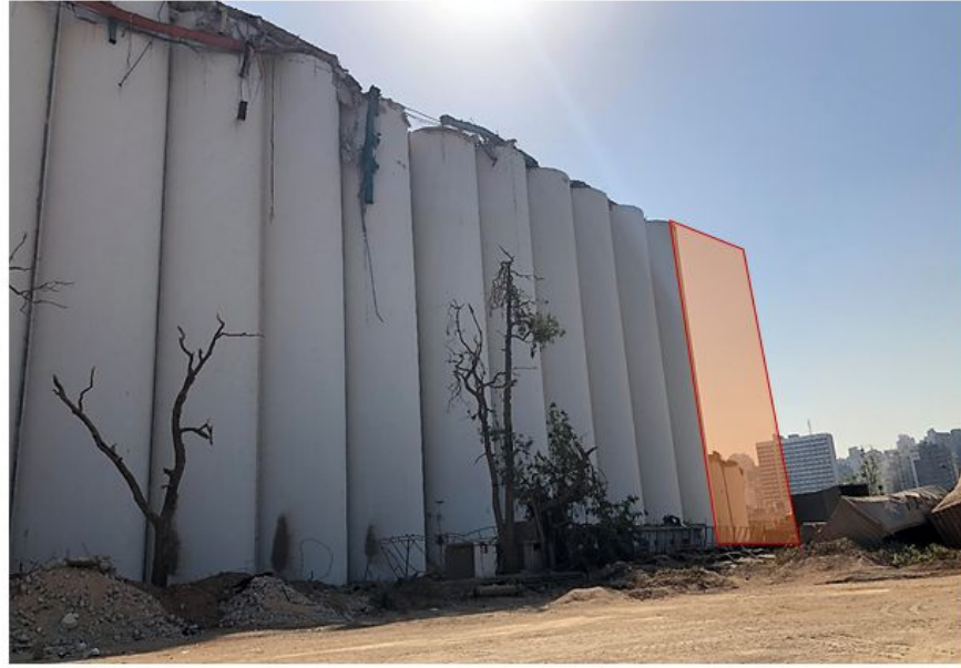
Figure 3.20. View of the third row of silos (of Phases I and II) on the opposite side of the explosion source. The location of the last two columns of silos (Phase III) is shaded in the image; those silos are completely destroyed and not visible in the picture. (33°54'5.31"N; 35°31'3.38"E).
