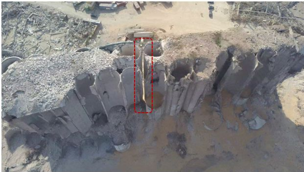
Figure 3.13. Image taken from a drone looking towards the west. The red box shows the interface between Phases I and II of the silo construction, where the construction gap was revealed by the damage.
